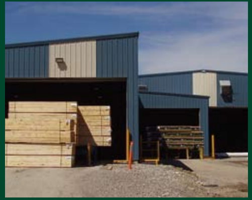
Spray Lake Sawmills 20,000 sq.ft. Treatment Plant and Building Addition
