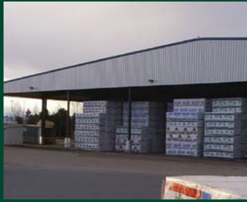
Mitsui Home Canada Inc. 38,000 sq.ft. Dry Shed Expansion
