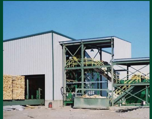
West Chilcotin Forest Products 20,000 sq.ft. Equipment Facility
